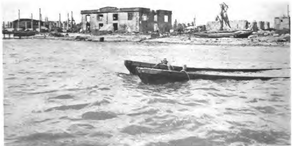
Top: The concrete house just north of Ormoc on Highway 2, after its capture by the 305th. Bottom: The Ormoc coast line as the sailors saw it.
